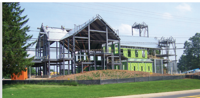
(Right) Construction of a new church for St. John the Apostle Parish, Leesburg
