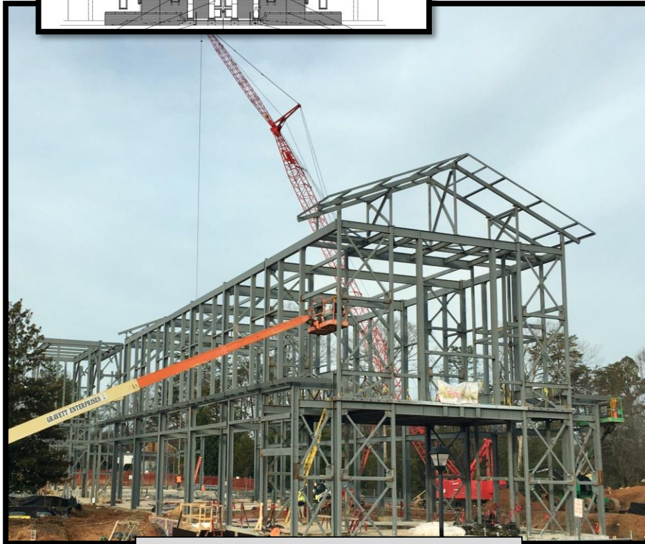
St. Mary of Sorrows Construction Underway
