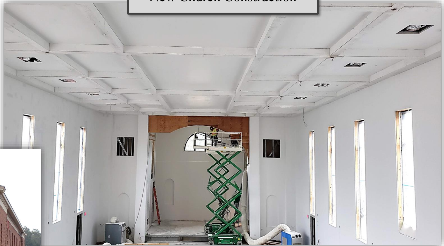
St. Patrick, Fredericksburg New Church Construction
